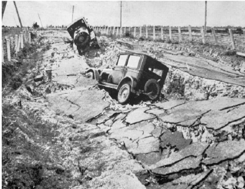
Figure 3.5 Liquefaction occurring under roadways will make them impassable except by all-terrain vehicles. Napier earthquake 1931 (GNS website).
