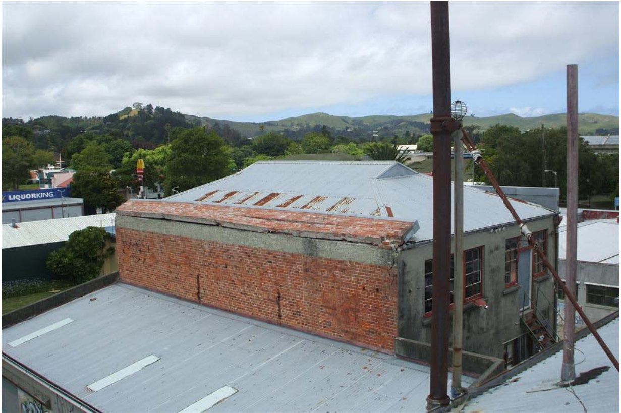
Figure 3: Indication of common mode of parapet failure parallel to the main street (noting unaffected roof below)
