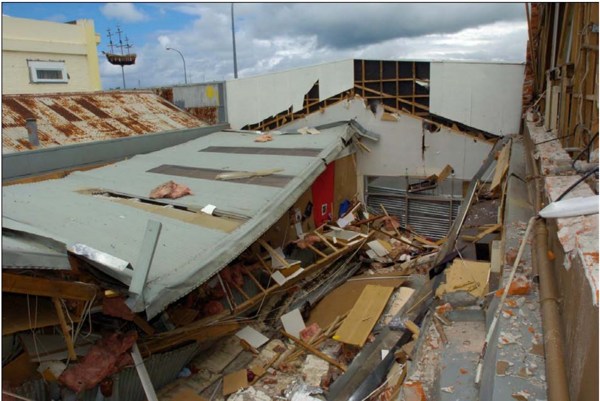
Figure 3: Indication of common mode of parapet failure parallel to the main street (noting unaffected roof below)
