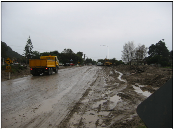
Figure 10: Transit NZ deployment of resources in Matata, May 20, 2005
